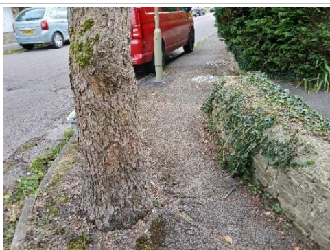
Figure 84: Footpath root damage near 18 Fox Close
