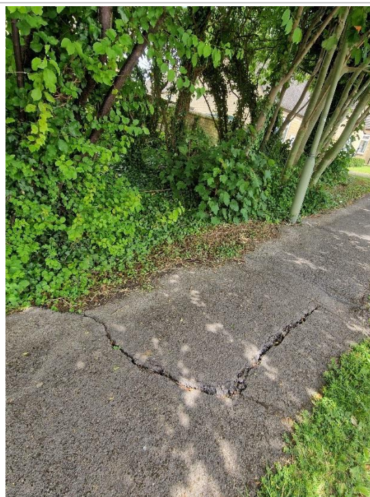
Figure 127: Crack in the surface of the footpath on Withers Way
