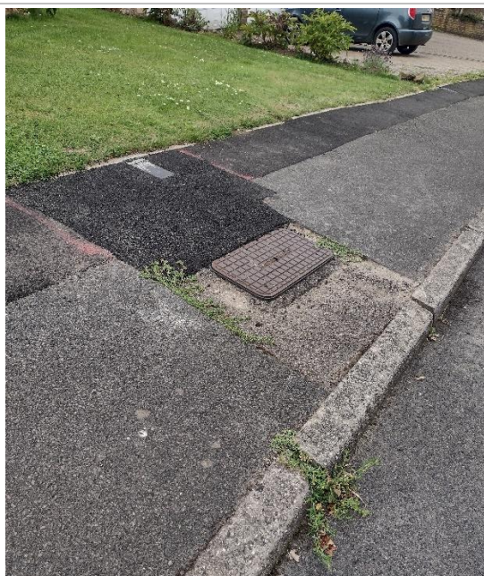
Figure 114: Protruding drain cover on footpath on Lewis Road
