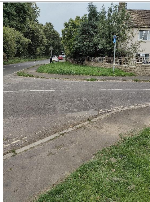
Figure 147: Dropped kerbs at the Tilsley Road / Churchill Road junction
