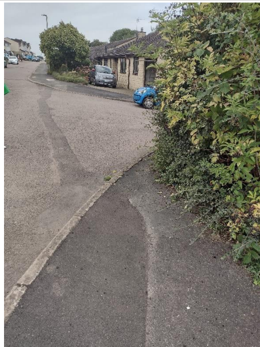
Figure 149: Break in northern side footpath between 33 and 35 Lords Piece Road. No dropped kerbs
